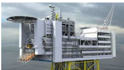
Enclosure for the Edvard Grieg project
