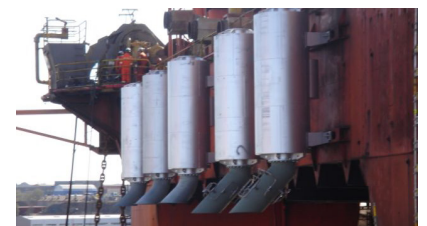
AISI 316 silencers on rig Transocean Searcher
