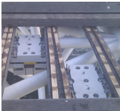
Installation under bridge 安装在桥下
