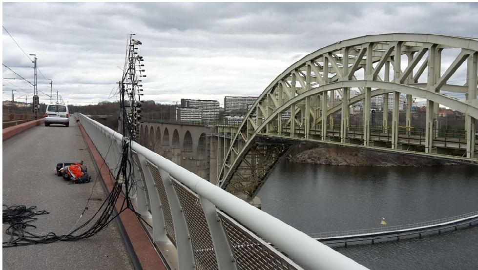
Figure 2 – Microphone array in front of steel bridge, Pos A.
